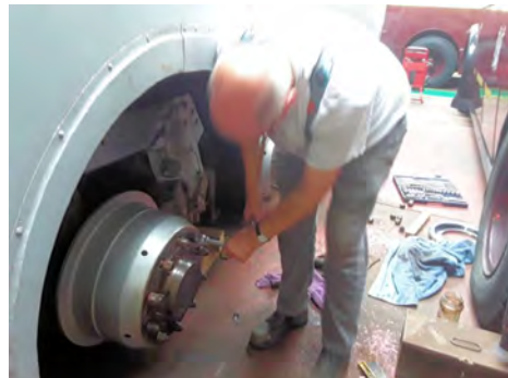
Jeff White fitting a refurbished brake drum to Cardiff 262. [Keith Walker]
