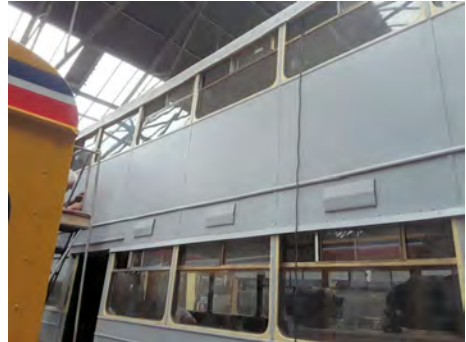
Cardiff 262's nearside double feather-edged beading being fitted. [Keith Walker]
